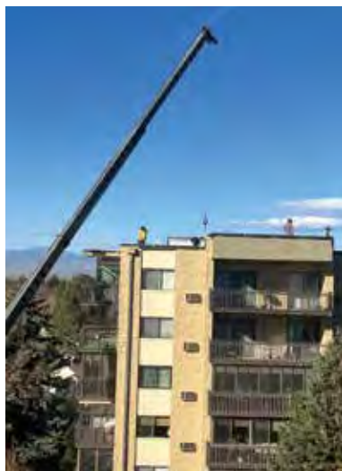
Crane offloads equipment from the B217 roof.
