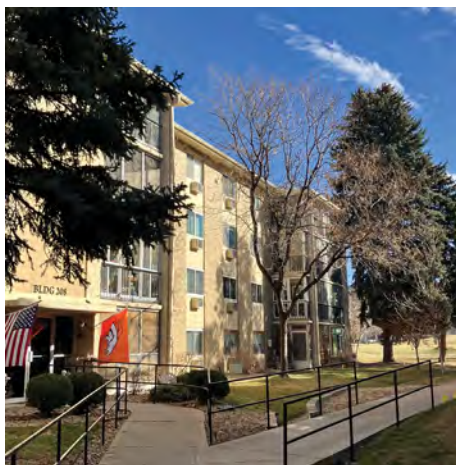
Building 208: One of the Alpha buildings where the roof will be replaced.
